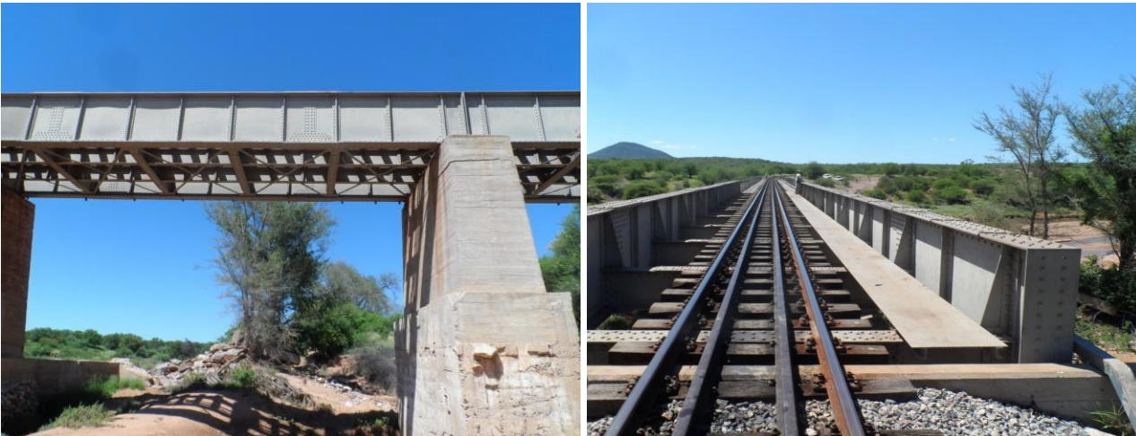
Figure 9- Railway bridge at Sand River
